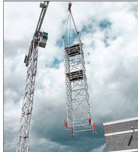
Crane eyes integrated in every frame
