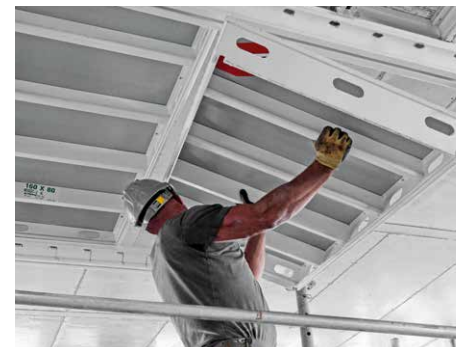
The ergonomic grip profiles facilitate installation, also from below.
