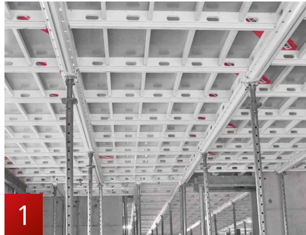
1 Drop-head-beam-panel method (FTE)
