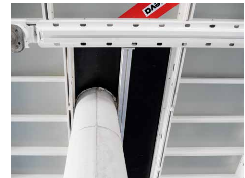
Fewer compensations saves time. Even uneven slab edges can be solved with a minimum of filler areas.
