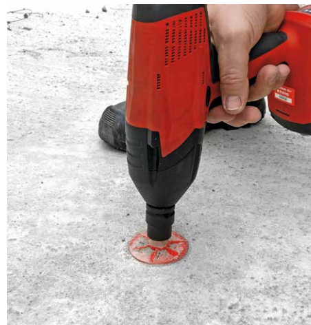
The anchor can be extracted by means of a power screwdriver, ratchet or open-end spanner (size 17).
