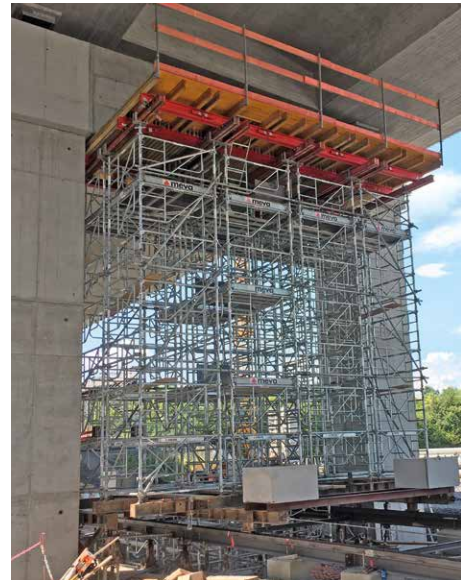
Motorway bridge near Heilbronn, Germany, MT 60 shoring tower, manoeuvrable on rails.
