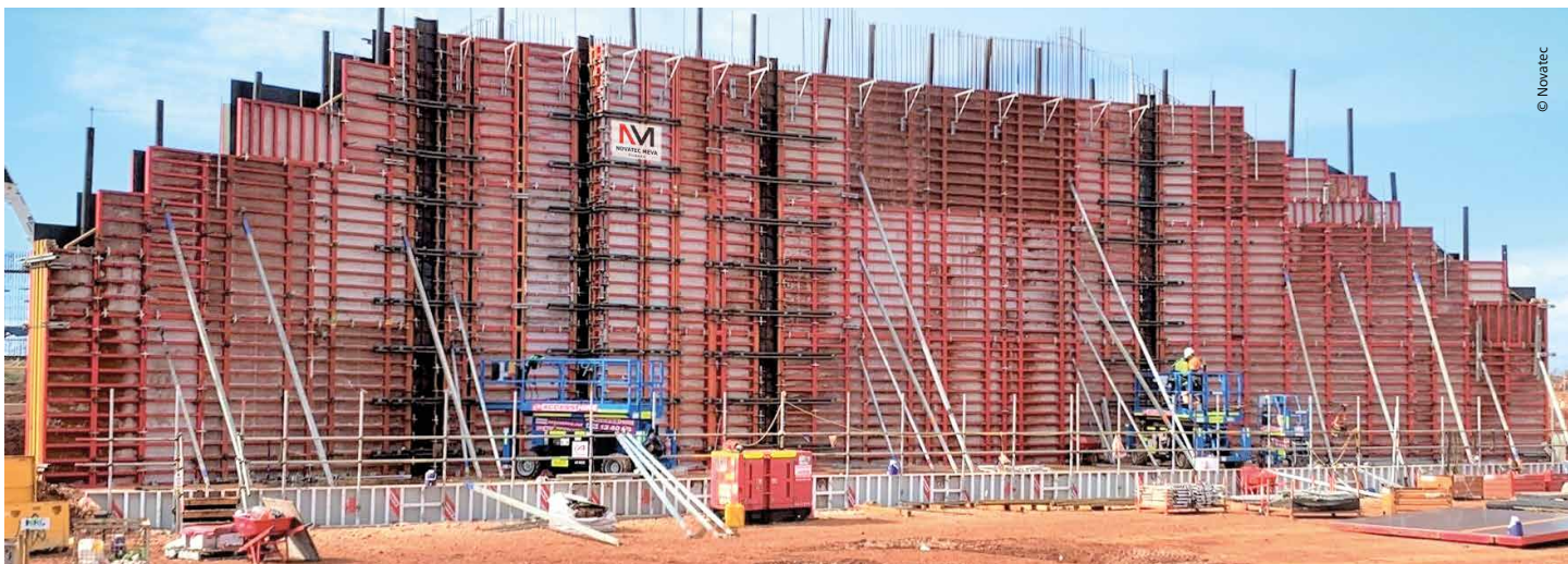
Abutments for a railway bridge, Pilbara mining region, Australia (Mammut 350).
