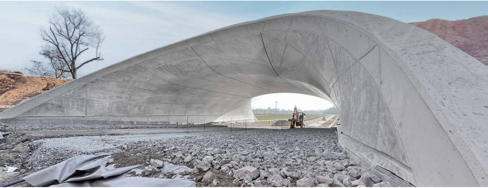
Combined cycle and pedestrian underpass in Mannheim, Germany, built with a clever combination of special and standard formwork.
