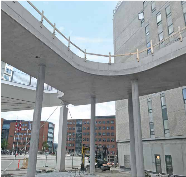
Rooftop garden at the CABINN hotel in Copenhagen, Denmark (MT 60 shoring tower, special formwork, AluStar and StarTec wall formwork).
