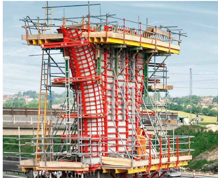
Bridge piers in Ferrybridge, England.
