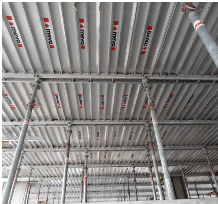
MonoDec slab formwork provides a high-quality concrete finish and consists of only three components.
