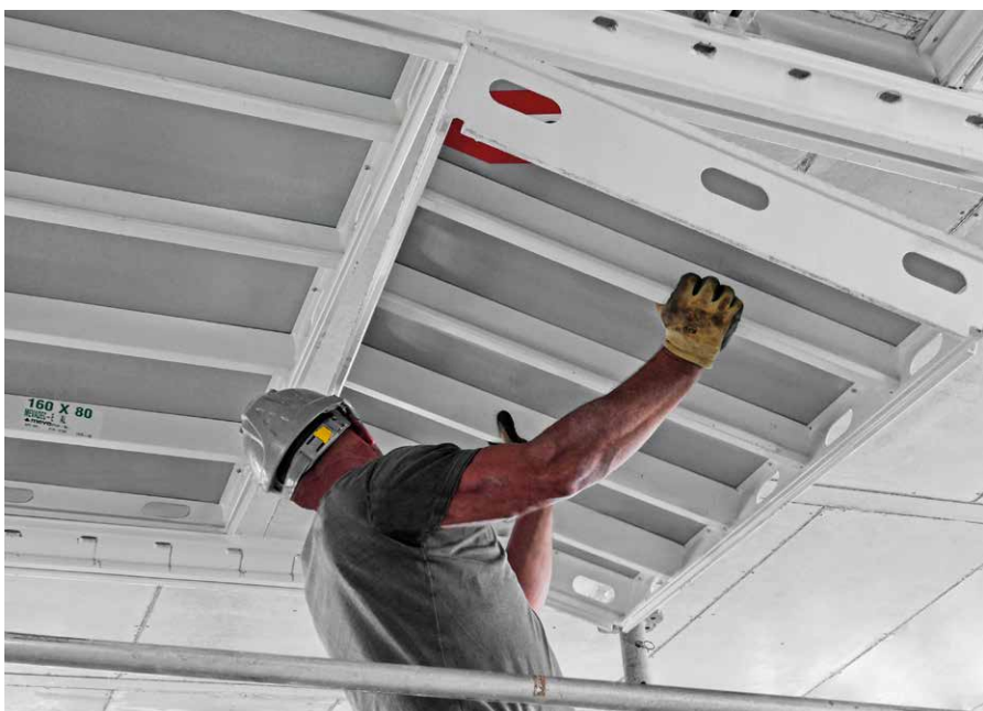
The ergonomic grip profiles make it easier to insert the panels from below as well.
