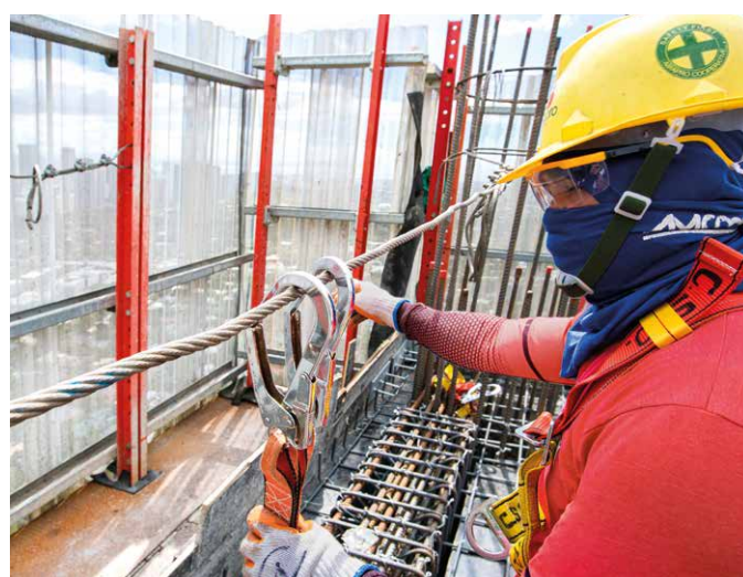
A worker from MBDI Construction unlocking after the MGS-H moved to the next level and provides full protection.
