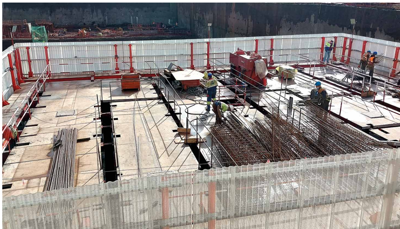
The fully enclosed unit protects workers from the elements and provides comfortable working conditions.
